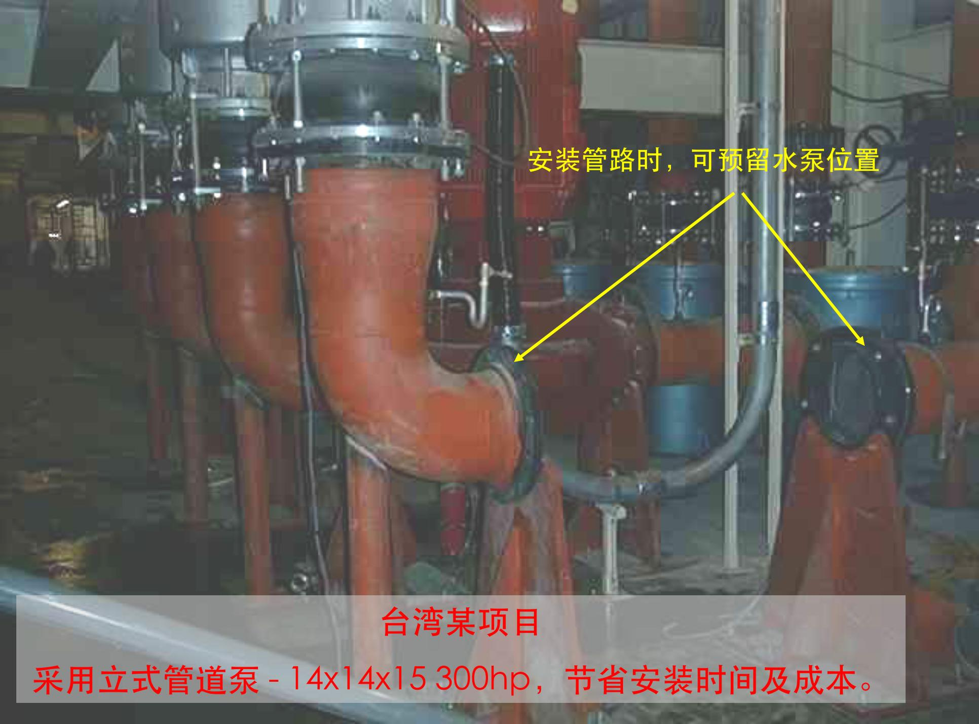
The image shows a complex industrial installation with multiple vertical pipes and pumps. The pipes are painted in a reddish-brown color, while the pumps are blue. The machinery is mounted on a metal frame. Two yellow arrows point from the text above to specific locations on the pipes, indicating where pumps can be installed.
